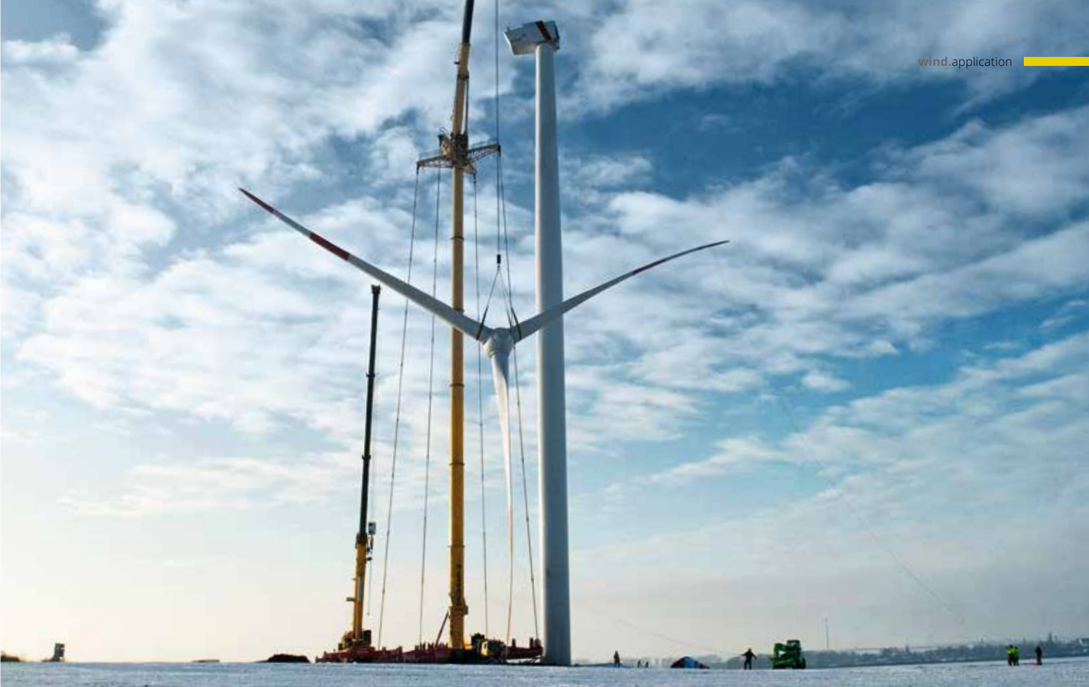
▲ Installation of an e.n.o. energy wind turbine in Saxony-Anhalt
