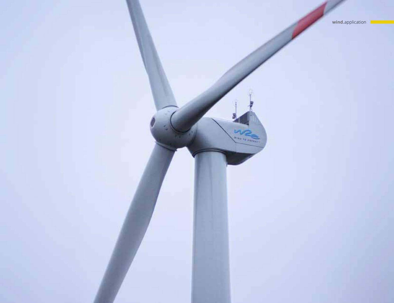
▲ With a tower height of 160 meters and a rotor diameter of 120 meters, the highest wind turbine in the world was the first in-house development from W2E. It was erected in Laasow, around 100 kilometers south east of Berlin in 2006.
