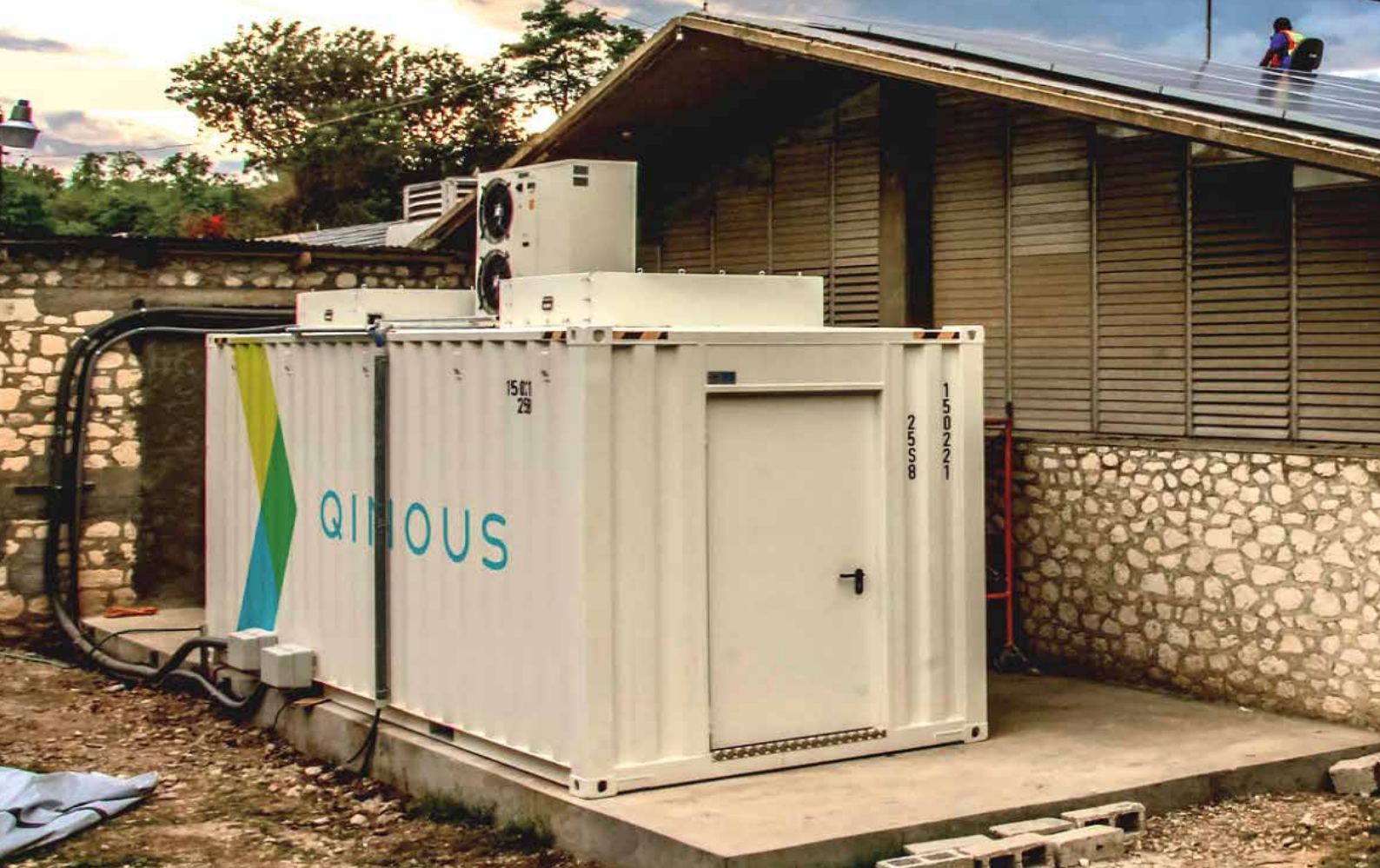
▲ Diesel PV battery hybrid system
