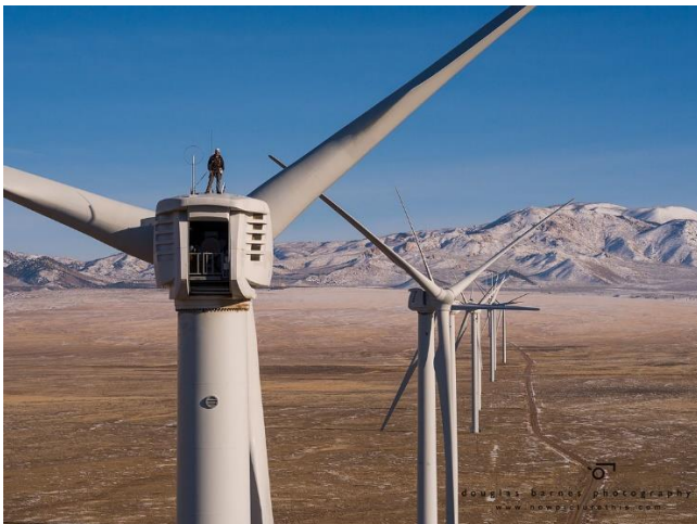
Milford I Windfarm in Milford/Utah
