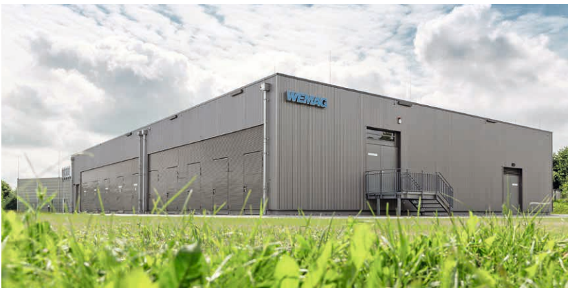
WEMAG's battery storage power plant in Schwerin-Lankow.
