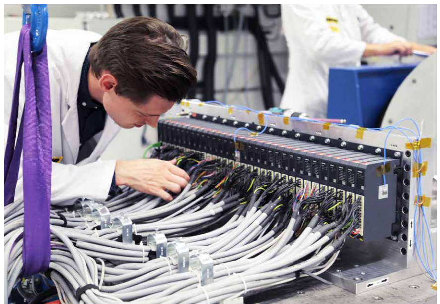
▼ The wiring is carefully checked to ensure that all connections have withstood the intense loads.
