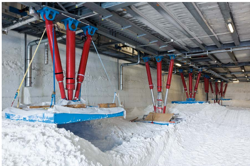
The Neumayer Station III, operated by the Alfred Wegener Institute, is supported by 16 stilts. Technicians regularly raise the station with a hydraulic lifting device to compensate for annual snow accumulation of about one meter.
