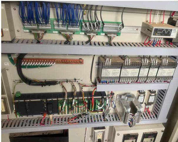
**Quick retrofit:** With pre-prepared stations and plug-and-play adapter sets, a controls retrofit can be completed in less than two days. This approach also minimizes installation errors. Pictured: The control system in the tower base, which also includes grid measurement.
