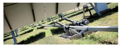
Electronically controlled tracking units of solar modules reduce the shadowing of modules at dawn and dusk, thus improving the overall output of the power station.
