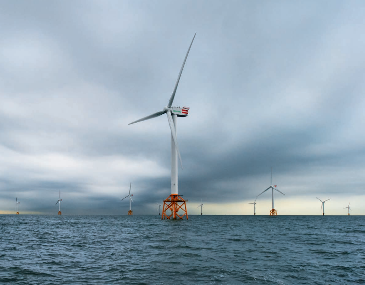
▲ 30 km off the Belgian coast: With an output of around 325 MW, the Thornton Bank wind farm is one of the largest of its kind in continental Europe.
