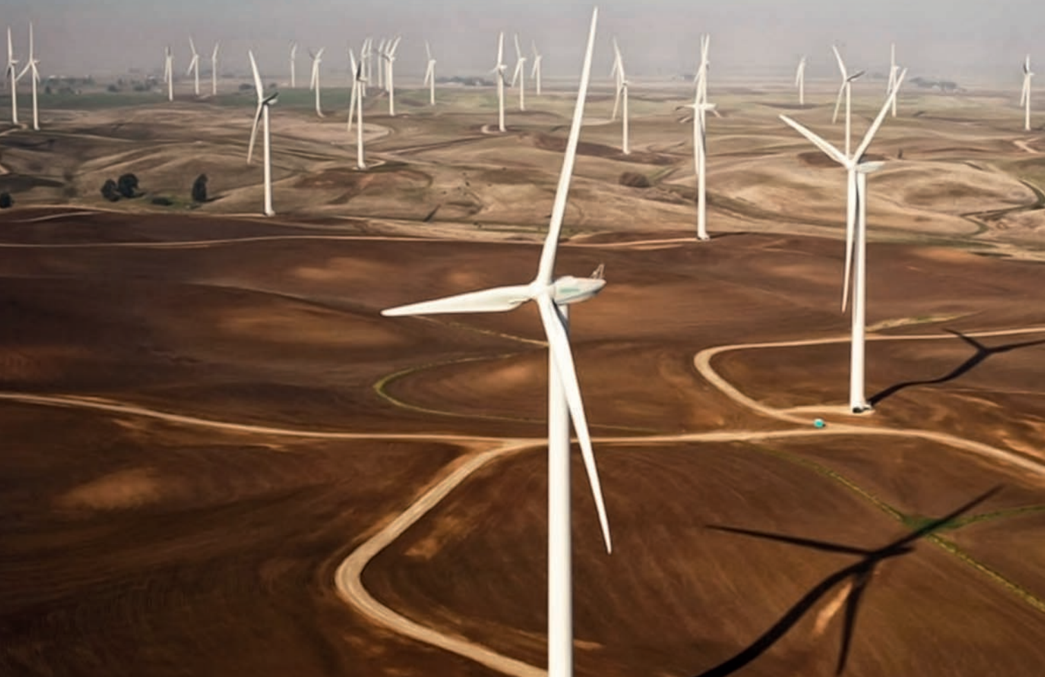
▲ Total output 355 MW: enXco Shiloh II, III and IV wind farm in Solano county, California (USA). This includes 175 MM92 turbines.
