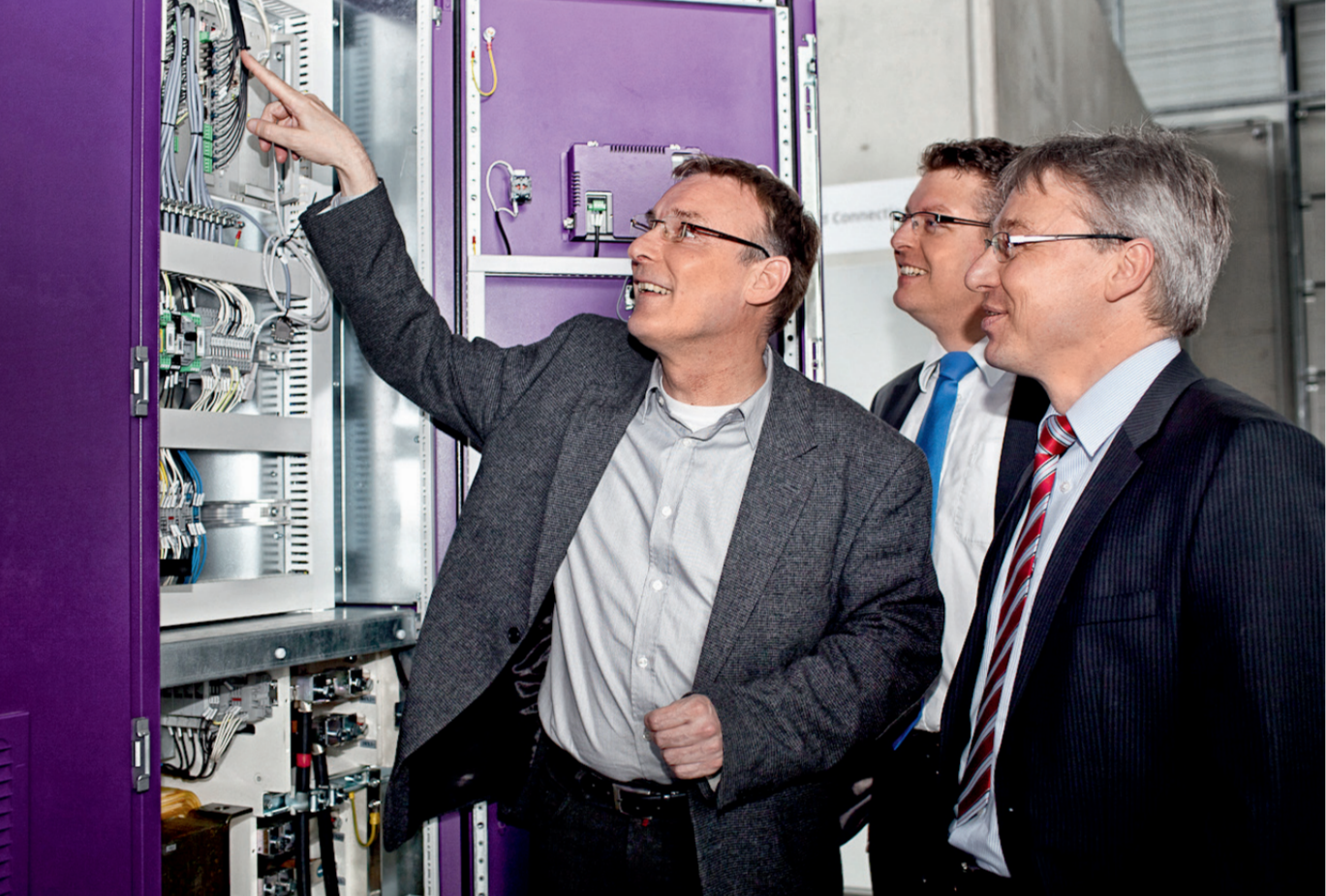
▲ Intelligent closed-loop control: Younicos-CTO Clemens Triebel explains to the WEMAG board member Thomas Pätzold the power plant management of the Younicos battery park.
