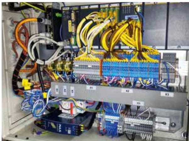
► Compact solution: The FEC is installed in the engine room and thus minimizes the cabling with retrofits.
