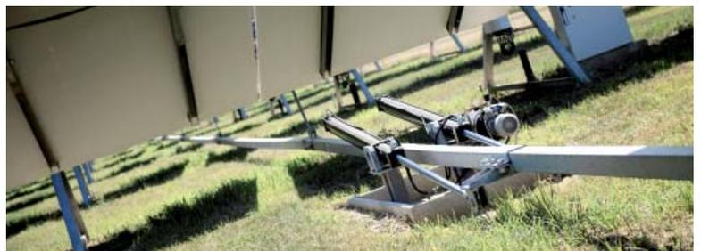
▲ Electronically controlled tracking units of solar modules reduce the shadowing of modules at dawn and dusk, thus improving the overall output of the power station.
