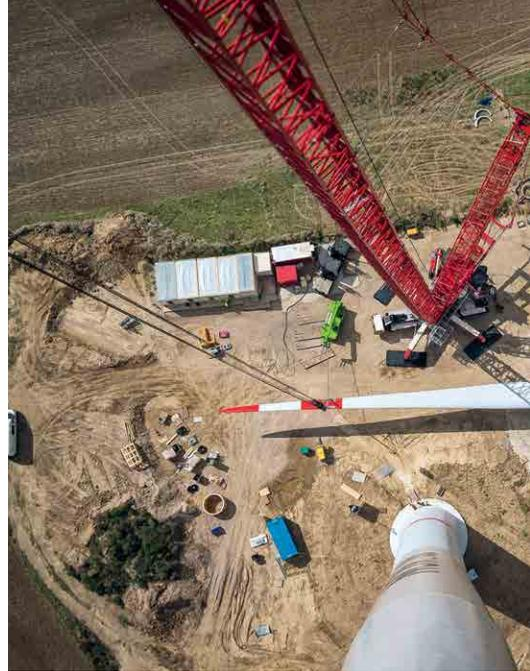
► of 3 megawatts. The hybrid tower of the wind power plant in Cracow (Mecklenburg-Western Pomerania) is not just manufactured from steel alone, but also has 1,500 tons of concrete in its lower section and 110 tons of steel tubing on the upper section. In this way it was possible to achieve in a safe and cost-effective way a nacelle height of 142 m instead of the conventional 94 m of towers made only from steel.
